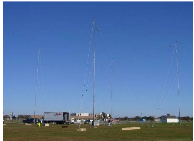
Figure 38. Completed small footprint eLoran system
