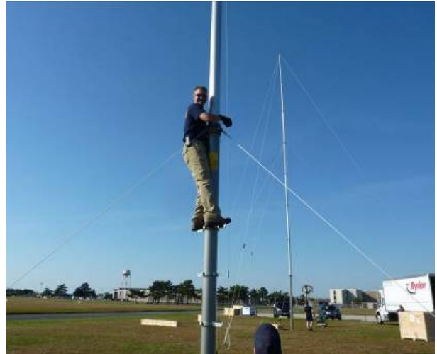
Figure 26. Extending the mast
