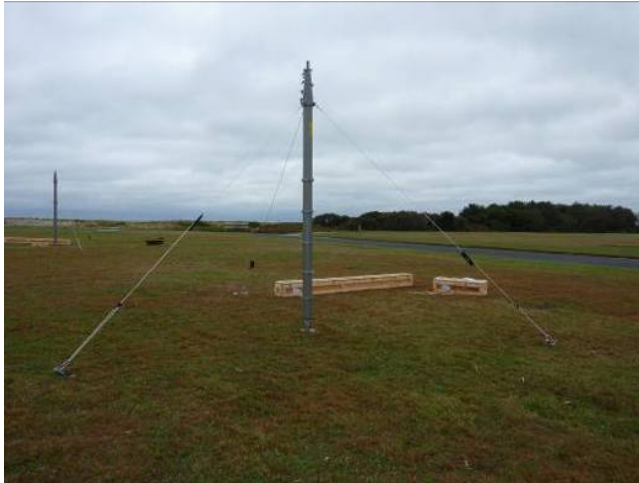
Figure 24. Antenna mast base section and guys
