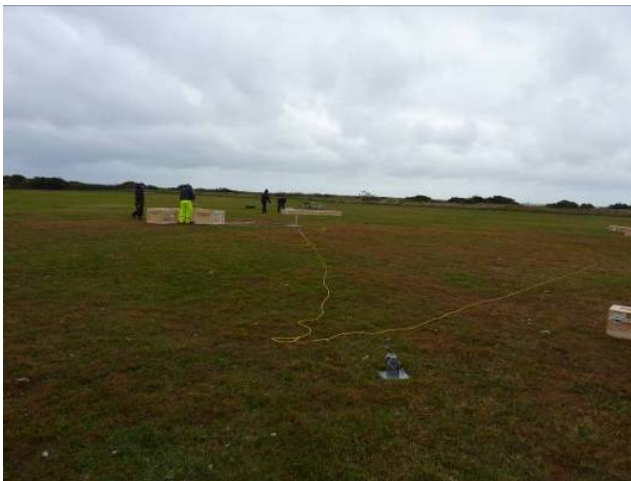
Figure 21. Marking the mast and anchor positions
