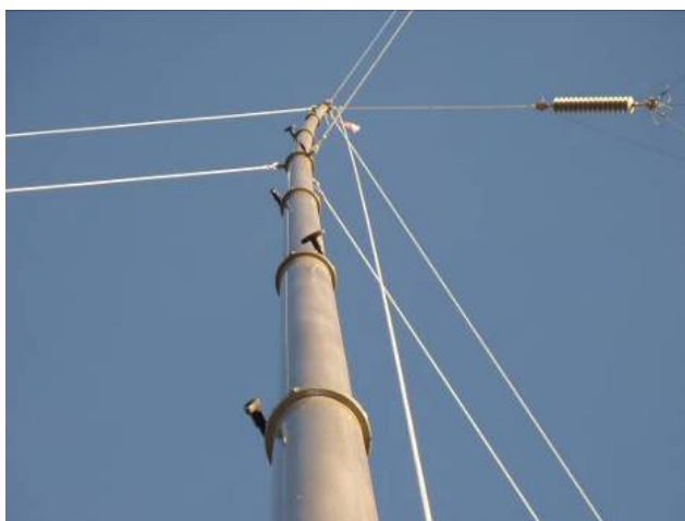
Figure 29. Strain on the mast due to the antenna
