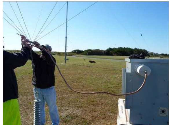
Figure 30. Connecting the antenna to the ATU
