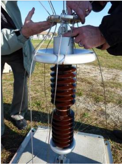
Figure 32. Oil-filled ceramic base insulator
