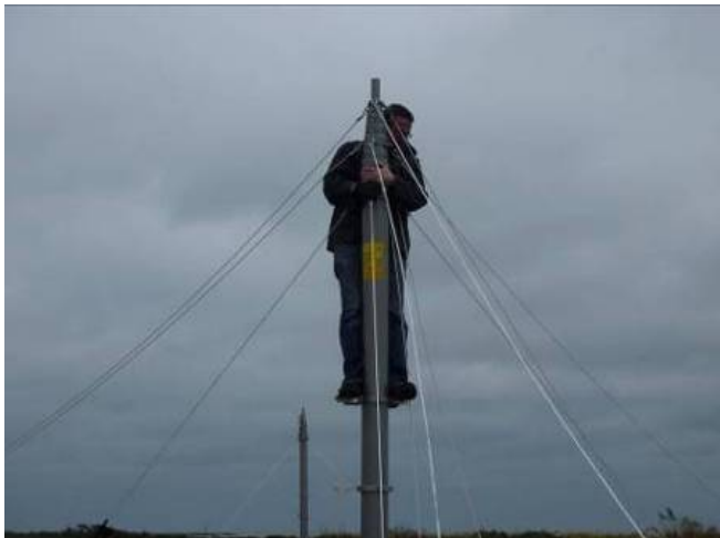
Figure 25. Positioning to extend the mast
