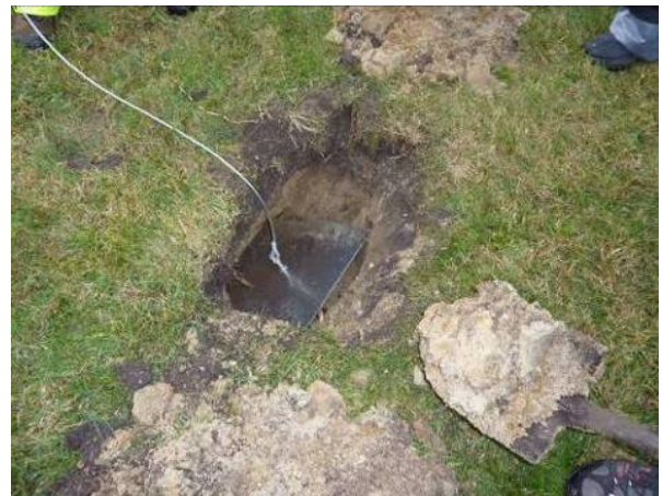
Figure 23. Outermost guy anchor plate
